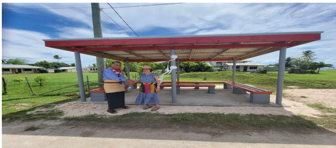
Bus Station at Ha'ato'u (Ha'apai) project, 2023
